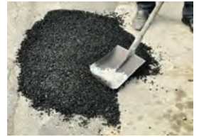
Repair both concrete and bitumen roads
