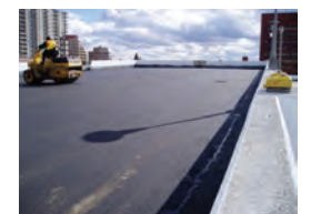
Cold patch used as waterproofing layer.
