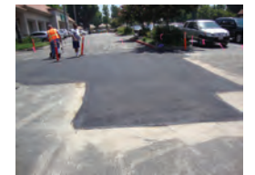
Parking lots repairs
