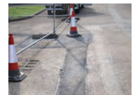
Trench reinstatements/ backfilling
